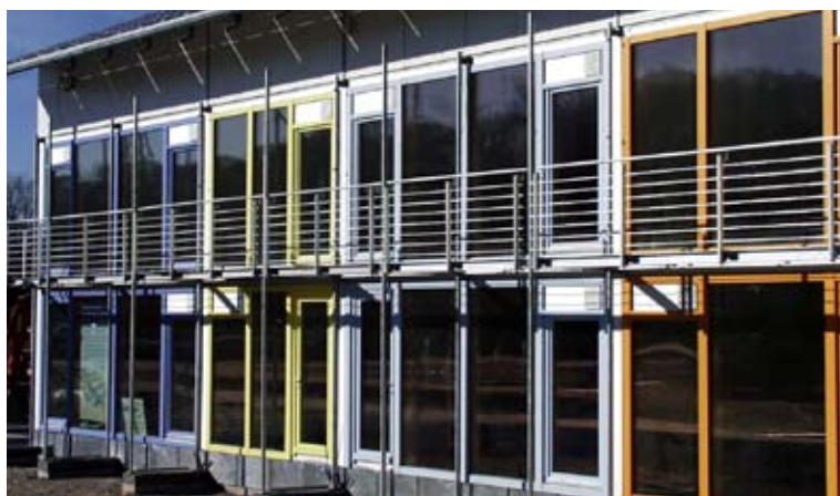
Drei3Holz solar facade for architect Disch, Freiburg 2000
