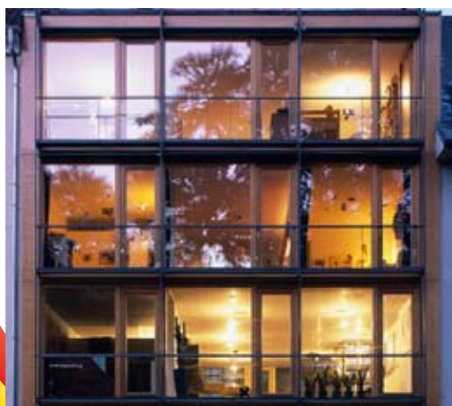
Drei3Holz solar façade for architects Altmann + Zimmer, Wiesbaden 2002 German Architecture Prize 2003
