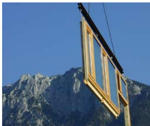
Transporting the pre-assembled facade elements
