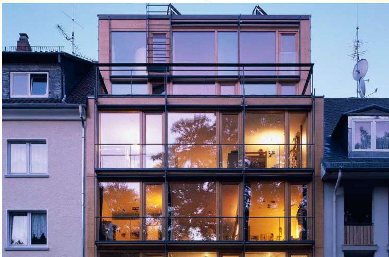
Drei3Holz solar facade for architects Altmann + Zimmer, Wiesbaden 2002, German Architecture Prize 2003
